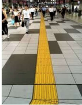
Figure 17. Braille bumps consisting of repeating raised patterns [22]
